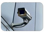
Figure 2: Bullet camera mounted on an exterior wall
